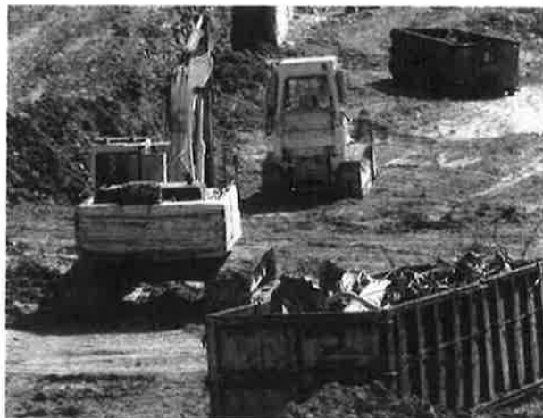
Construction waste should be collected in designated waste collection areas on-site, such as metal dumpsters.
